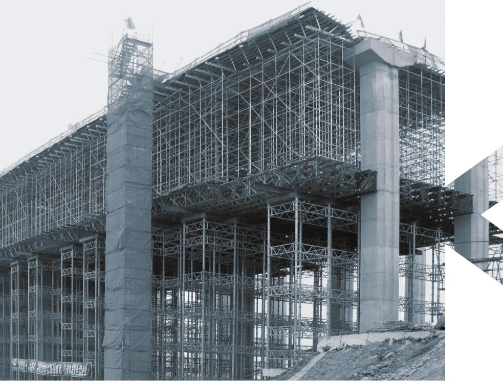
**Guilong Highway in China.** One million cubic metres of SPS, Duralok and SBS 135 material were used for the construction of the 12 km long Highway in the Guizhou Province. Special designs of shoring had to be done for the project.
