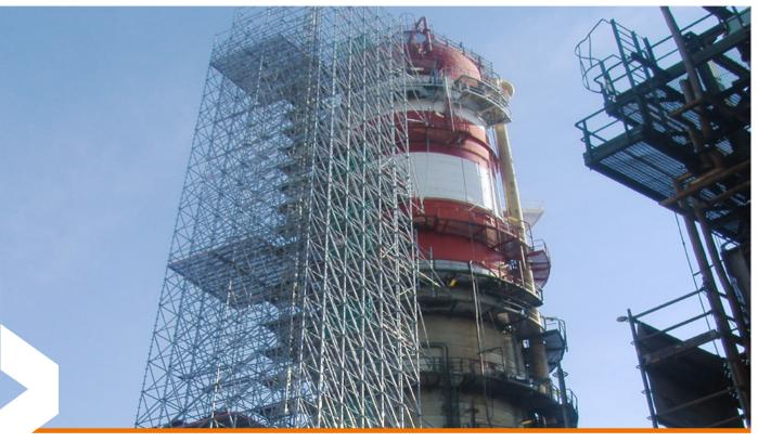
**Repsol Refinery in Spain.** The assembly of the 90 metres high RINGSCAFF scaffold for sandblasting work at the refinery in Tarragona was a real statical challenge.
