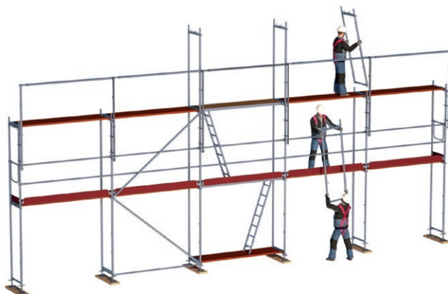
Figure 30: Assembly of the scaffolding level in the protection of the mounting safety guardrail
